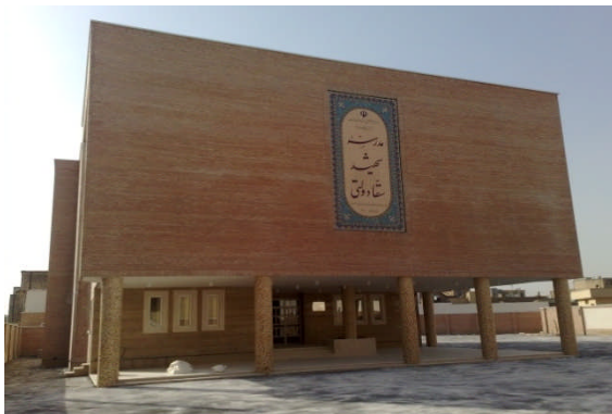
Picture1 : The Constructed Primary School
